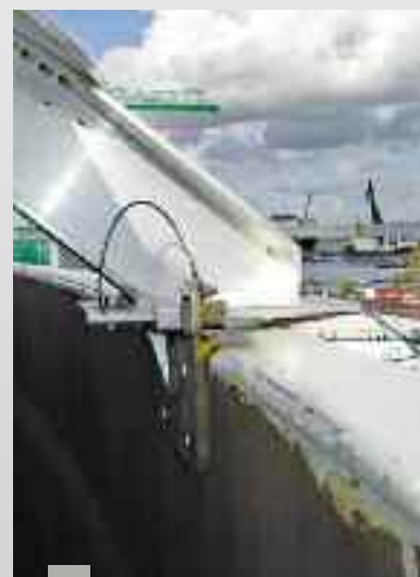
Sliding dome support with anti static wire
