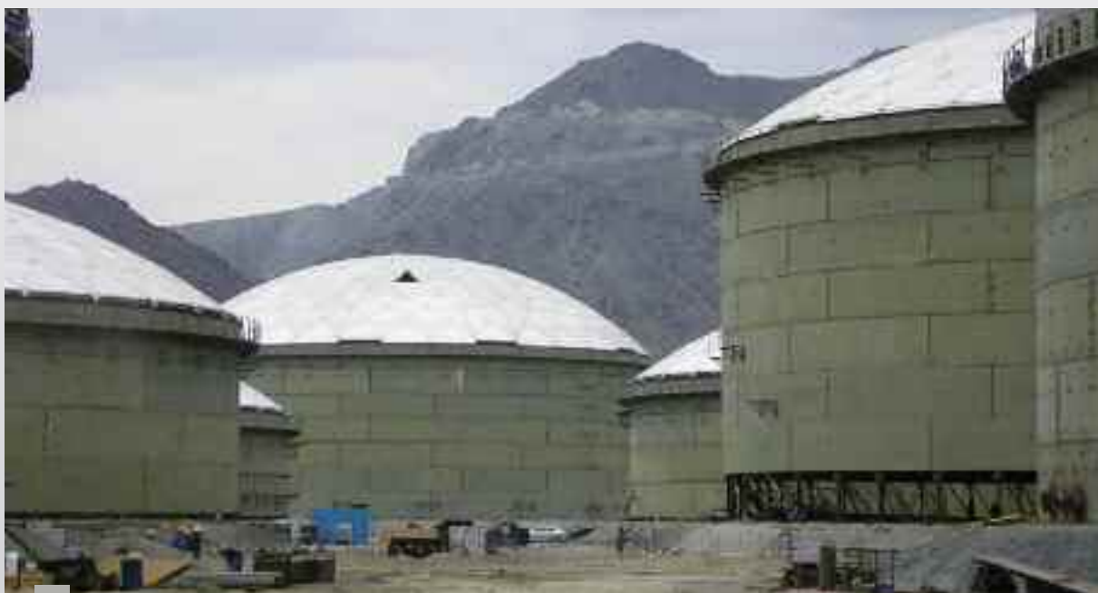
Vitol UAE domes under construction
