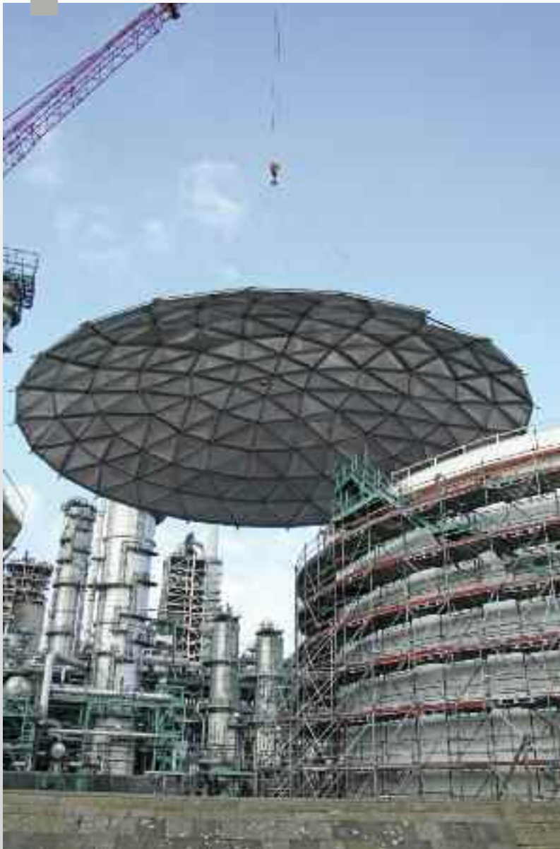
ExxonMobil refinery dome lift, The Netherlands
