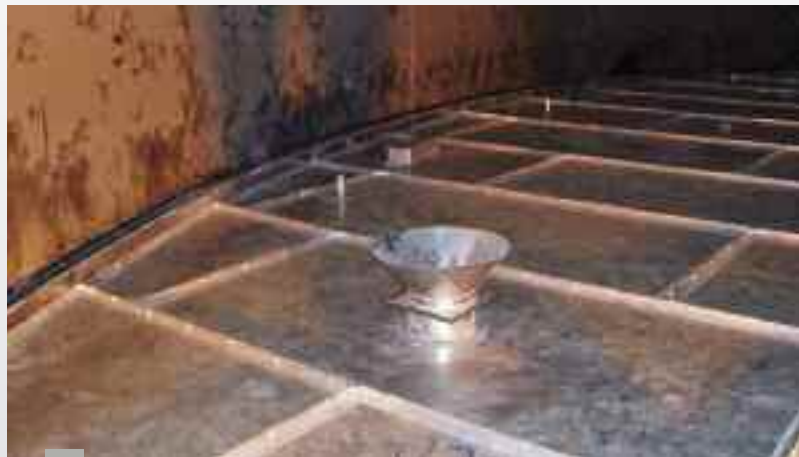
Top view aluminium full contact IFR, showing gauging and sampling funnel
