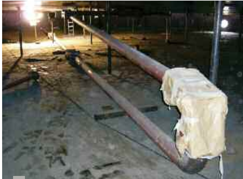
Drain line with Drainmasters during tank painting program
