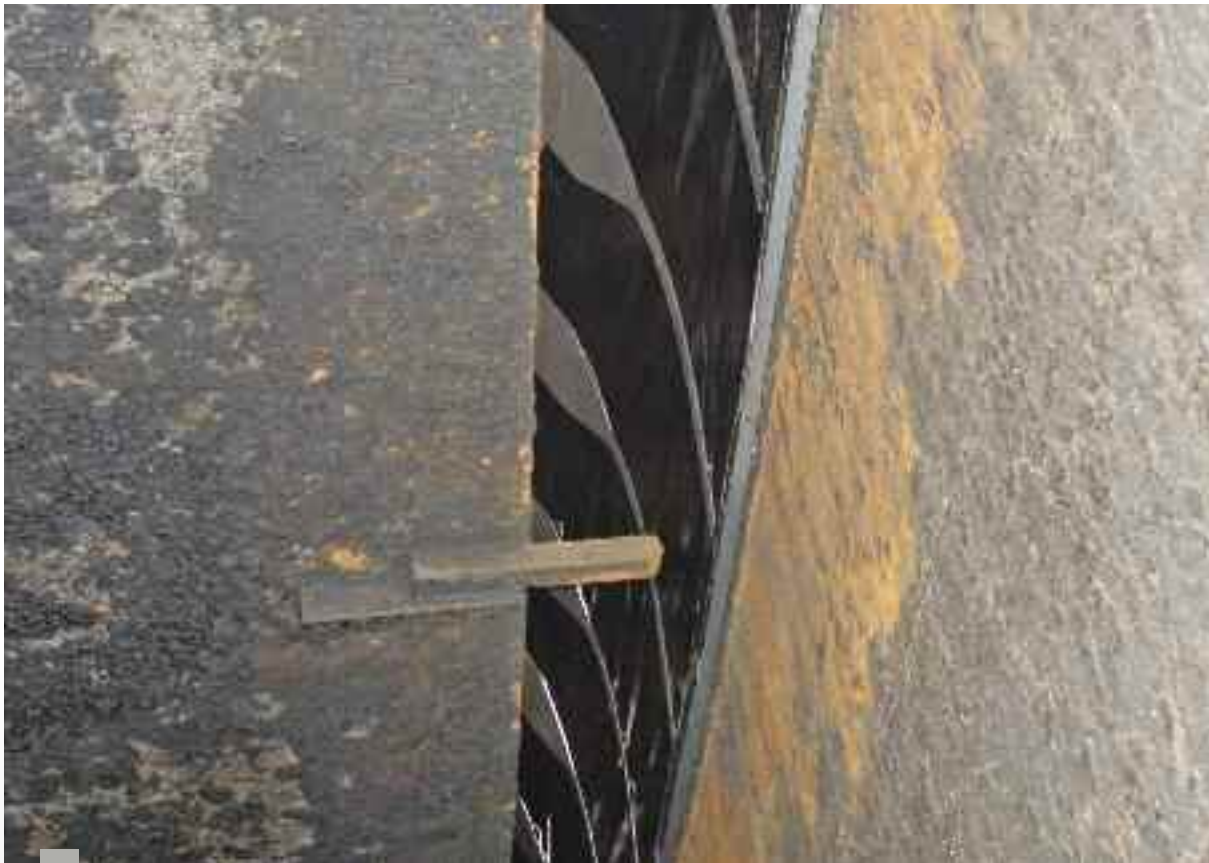
CTS30 BP CTS30 liquid mounted primary seal with integral wax scraper, bottom view
