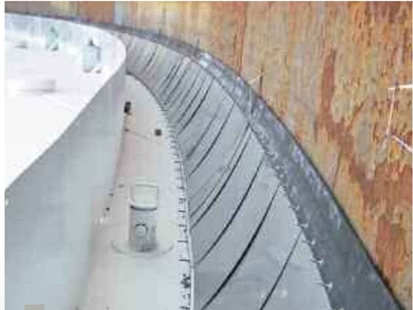
CTS20IT (Integral Tip) secondary tank seal
