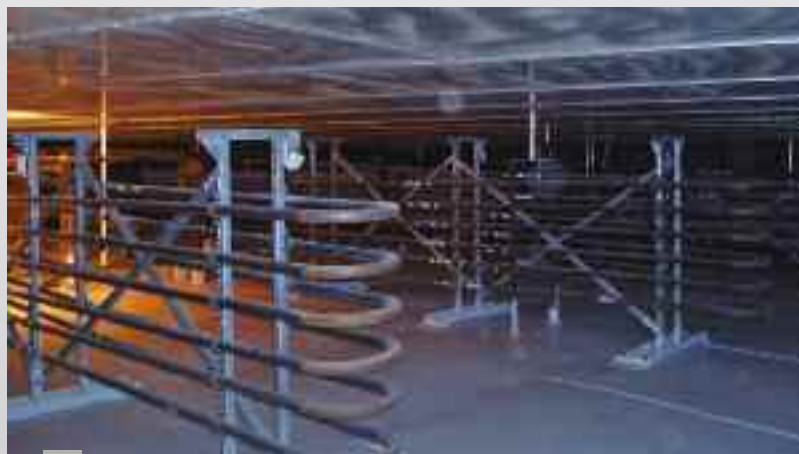
Bottom view aluminium full contact roof
