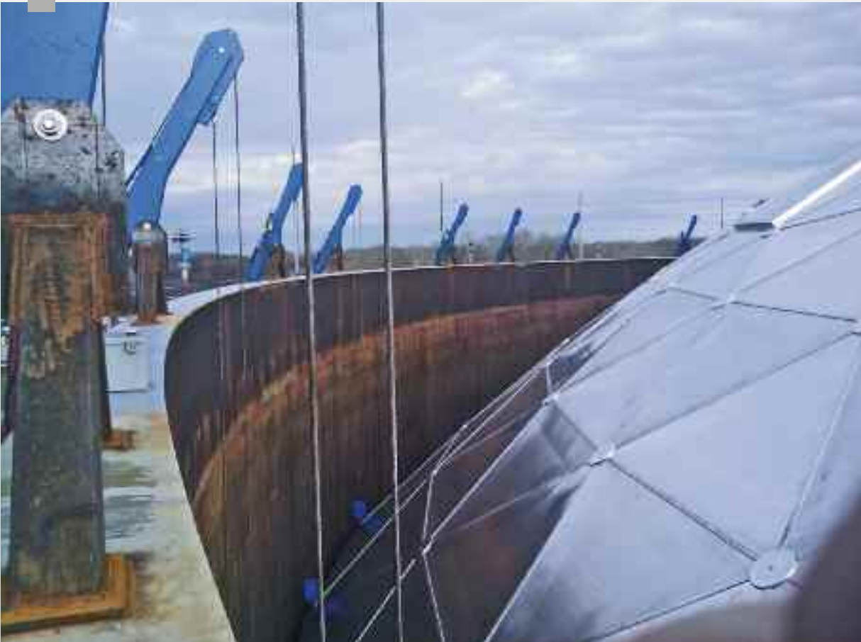
Dome lift using grip hoists at OMV Vienna, Austria
