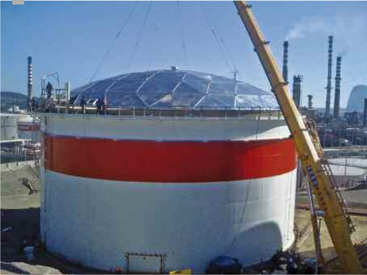
Dome lift by crane at CEPSA Algeciras, Spain
