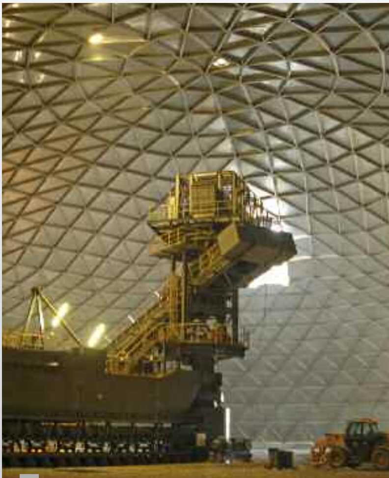
Bulk storage dome, interior view after completion
