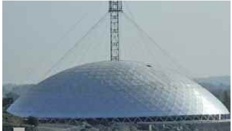
105m diameter dome under construction by CTS
