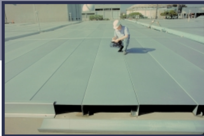
Vlakke afdekkingen voor bezink basins, County Sanitation District, Orange County, USA.
