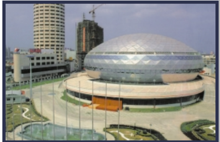
Shanghai International Gymnastics Center, Shanghai, China.
